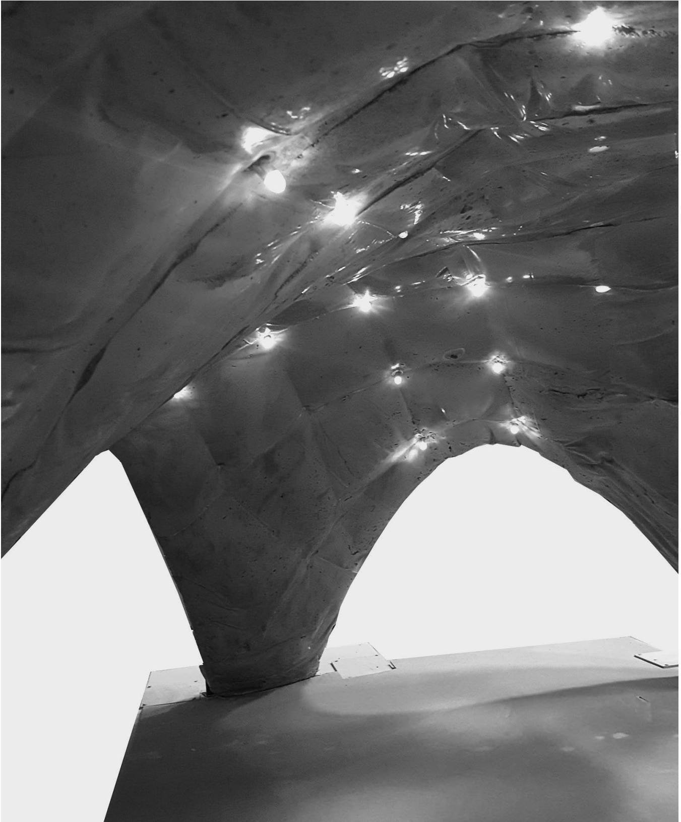
Saliklis-Olsen Interdisciplinary Studio: Interior quilted texture through plastic stretched over wood waffle grid by Cordova, Da Silva, Franco, Roth.
