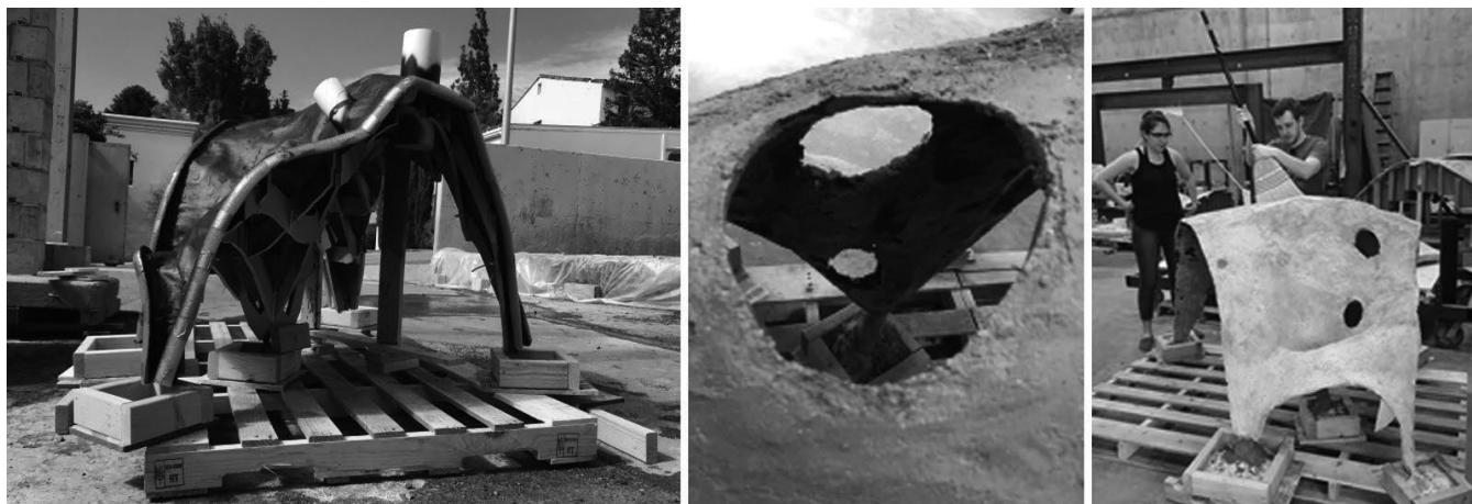
Figure 3: Saliklis-Olsen Interdisciplinary Studio: Material savings achieved through geometry, formwork and ultra-thin concrete by Berridge, Cano, Choy, Ojalvo.
